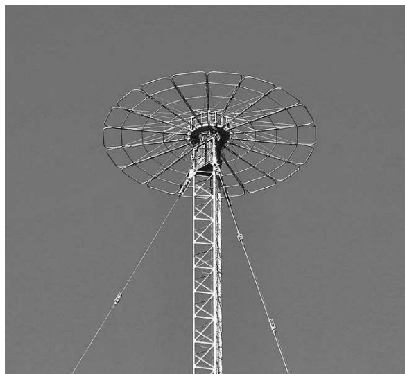
An example of a capacity hat, as used at many ABC AM broadcast sites operating on the lower end of the band. (Wikipedia)
