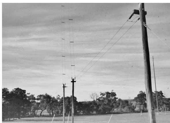
Pole supported open wire feed line.
