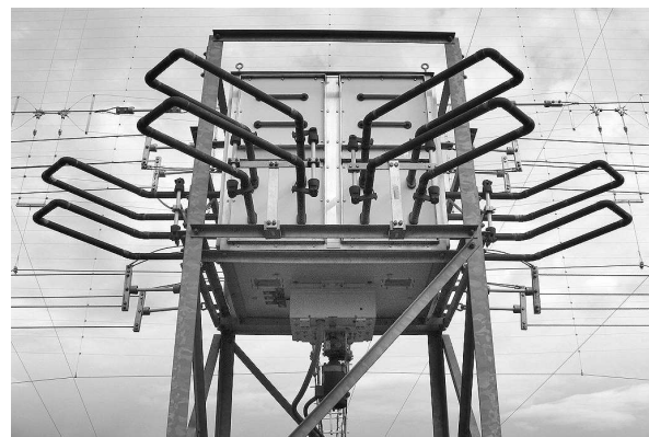
Part of an antenna slewing network at Radio Australia Shepparton.
