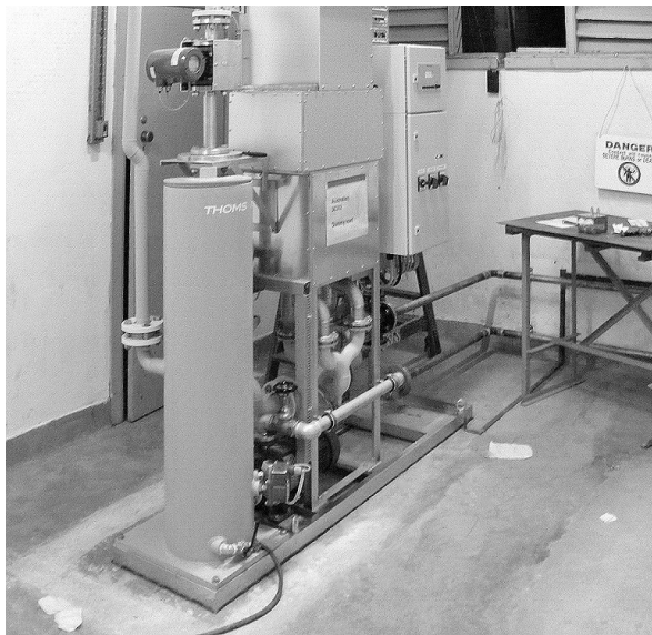
200 kW RF dummy load as at 2007.
